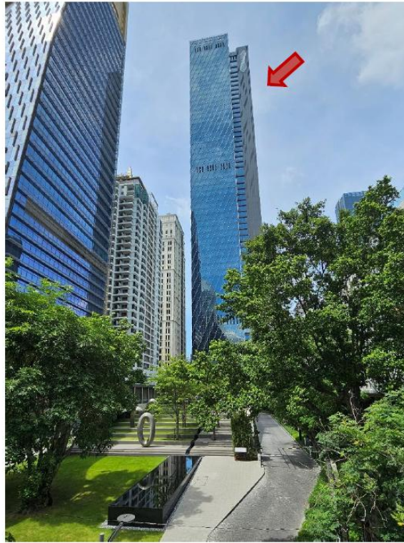
ONE CITY CENTRE BUILDING
